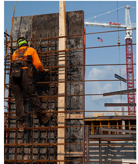
[below] Workers installing re-bar
